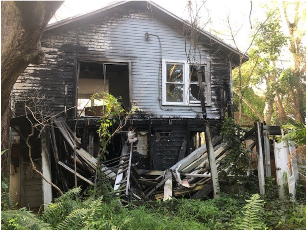
FAÇADE OF THE SUBJECT STRUCTURE
