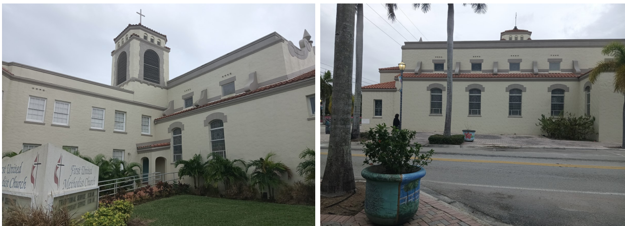
FAÇADES OF THE SUBJECT CHURCH
