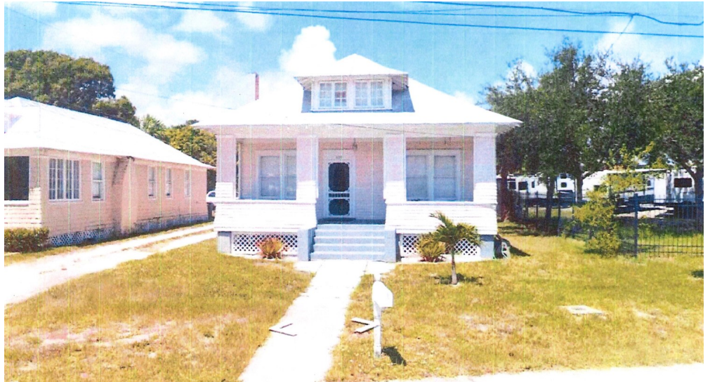
SUBJECT RESIDENCE - FRONT FACADE
