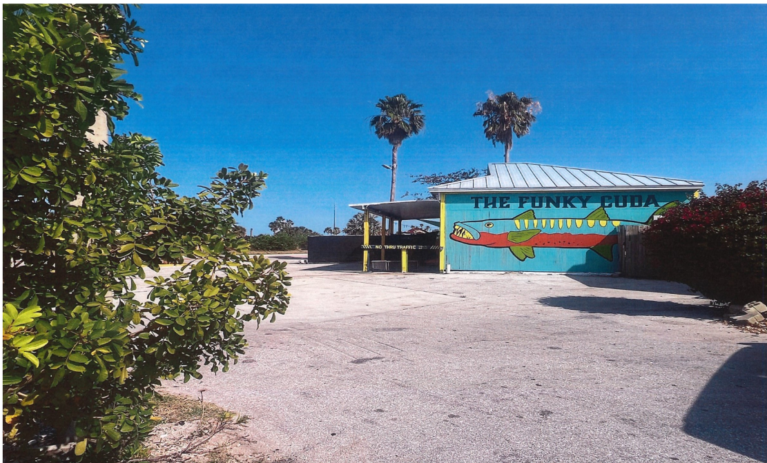
EXISTING FAÇADE, NORTH OF THE PROPERTY
