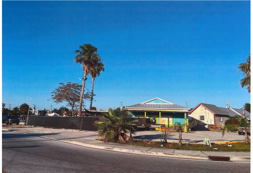
SUBJECT STRUCTURE - FRONT FACADE
