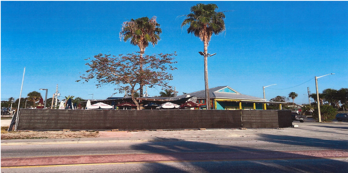
EXISTING FENCE, EAST SIDE OF THE PROPERTY
