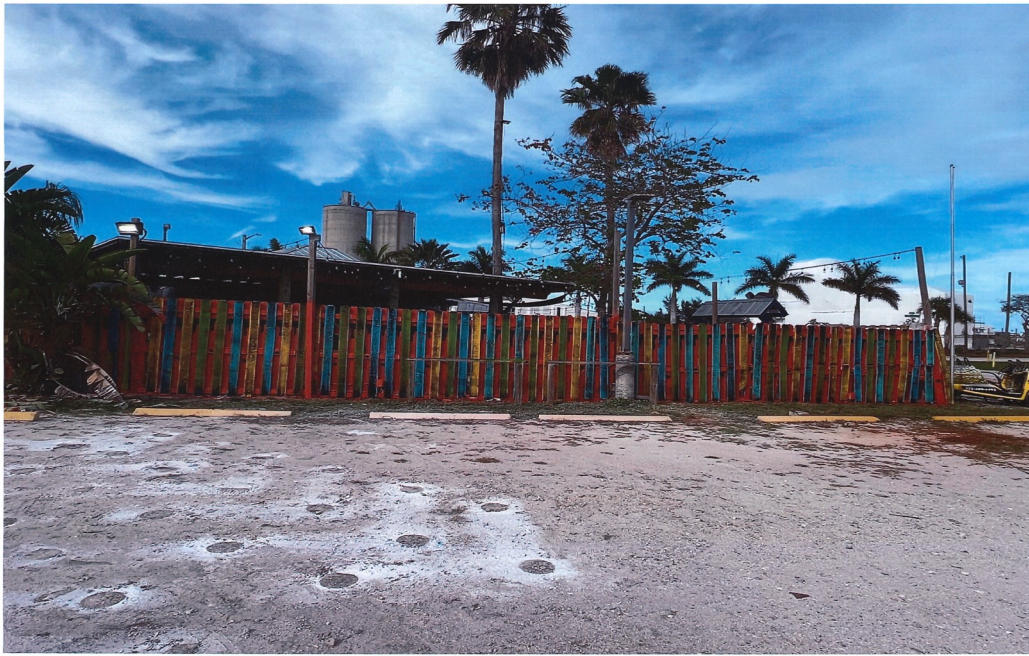
EXISTING FENCE, SOUTH SIDE OF THE PROPERTY
