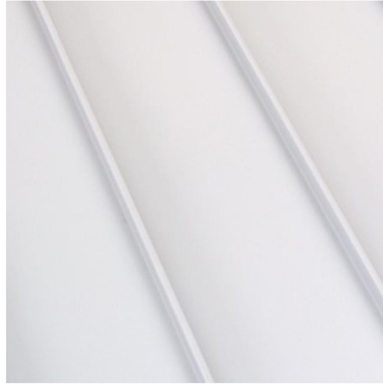
1 STANDING SEAM METAL ROOF
