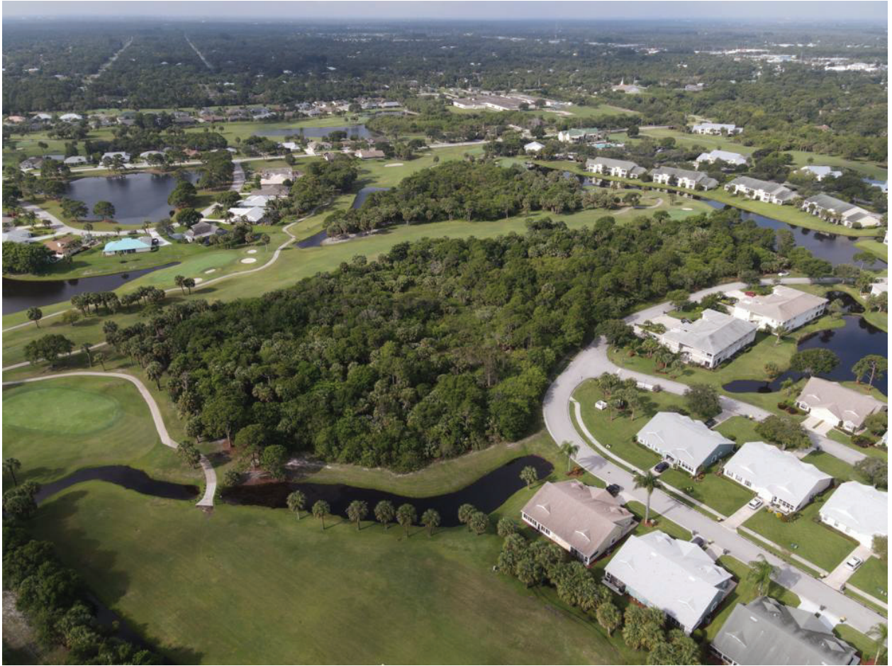
Photograph #2: View from North-East
