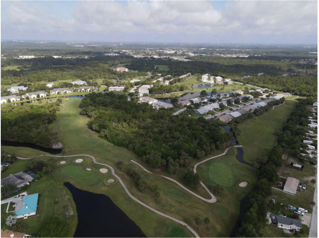
Photograph #4: View from South-East
