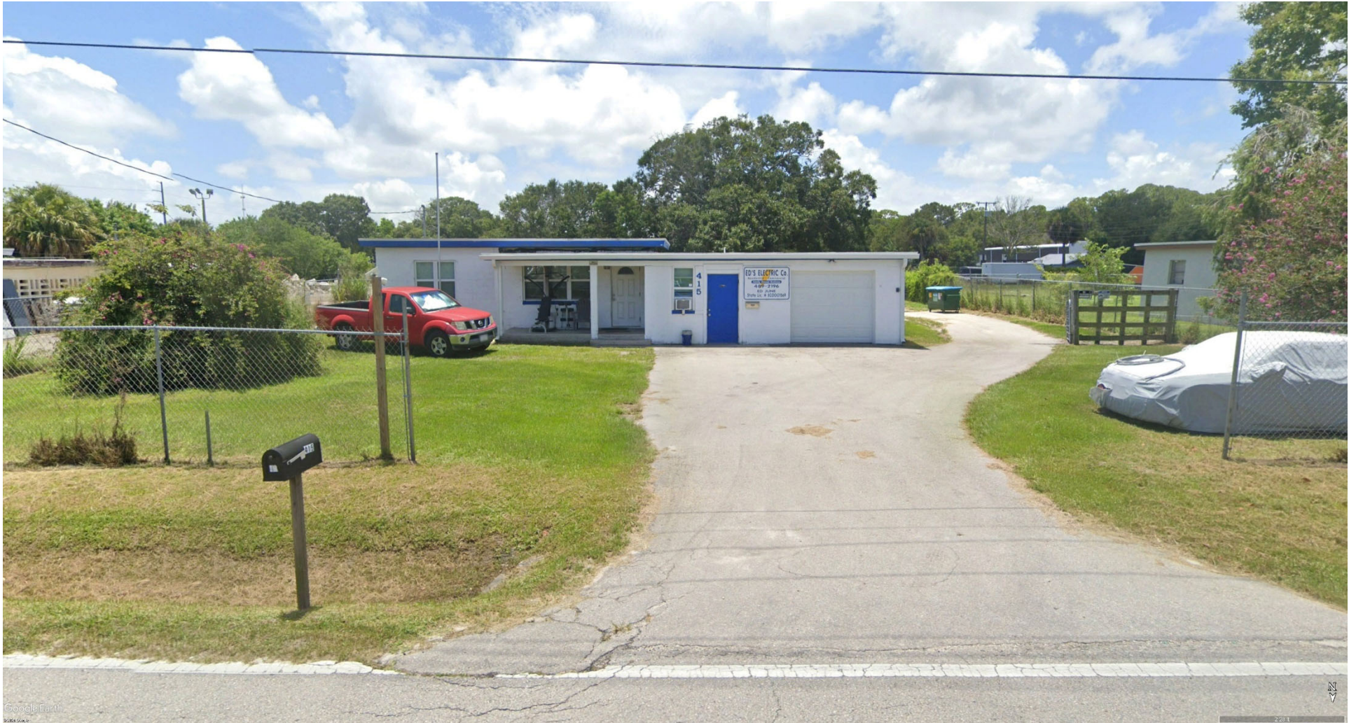
Photo 3 - Repair Services Parcel ID: 3403-502-0010-000-0
