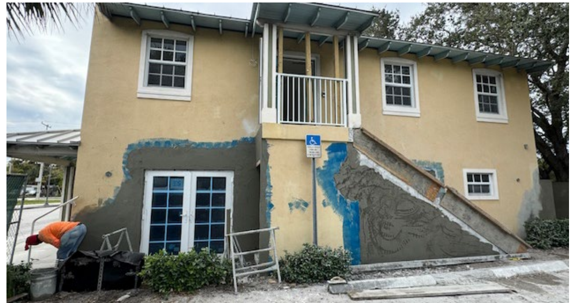
East Elevation: The new design features a canopy over the main entrance, along with a reoriented staircase.
