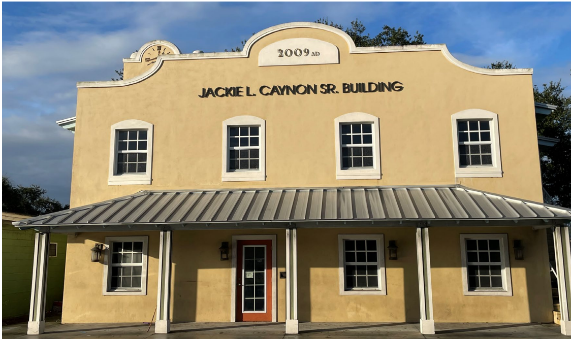
South Elevation: The existing door will be closed to create a wall.
