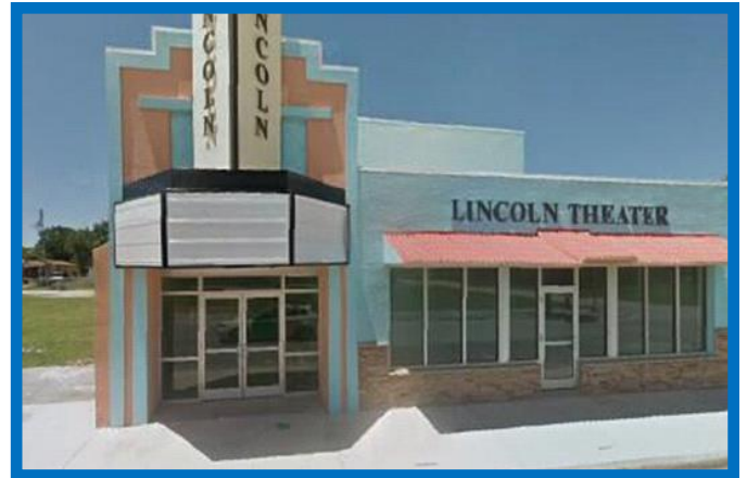
Historic Lincoln Theater Avenue D – Lincoln Park Neighborhood
