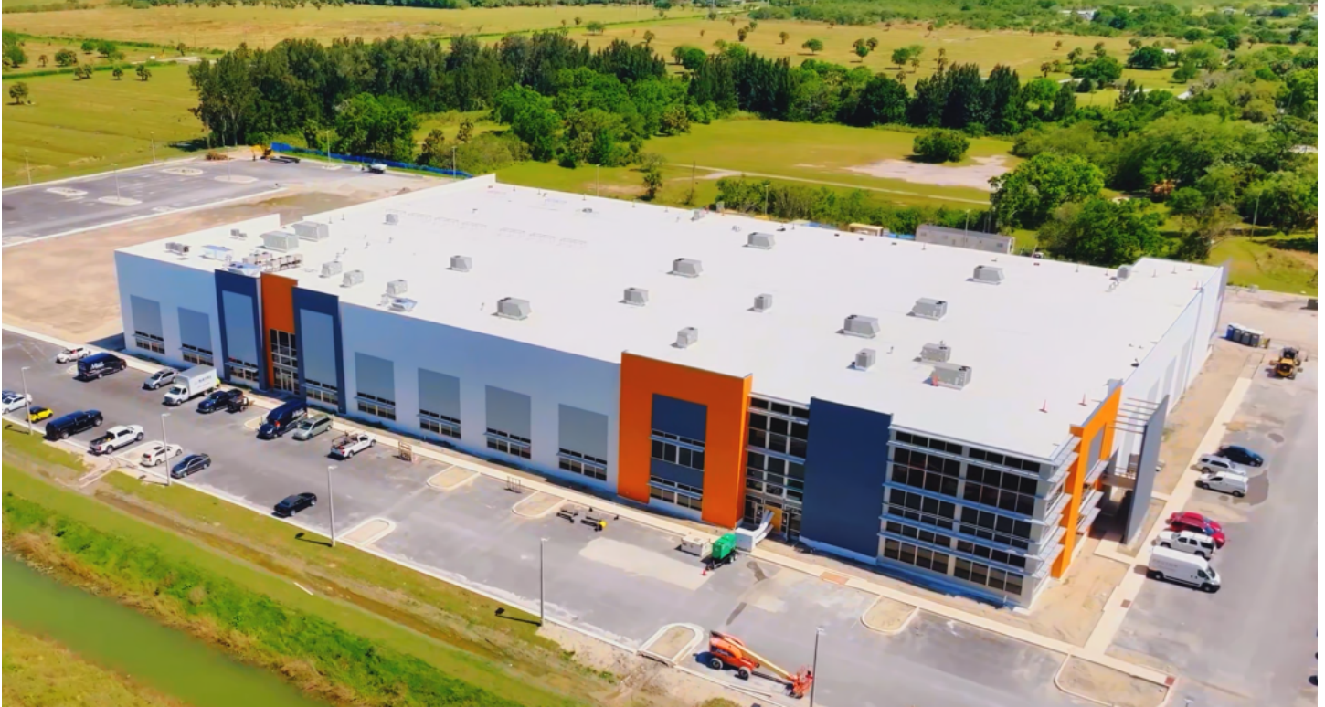
Treasure Coast Food Bank under construction, Spring 2025
