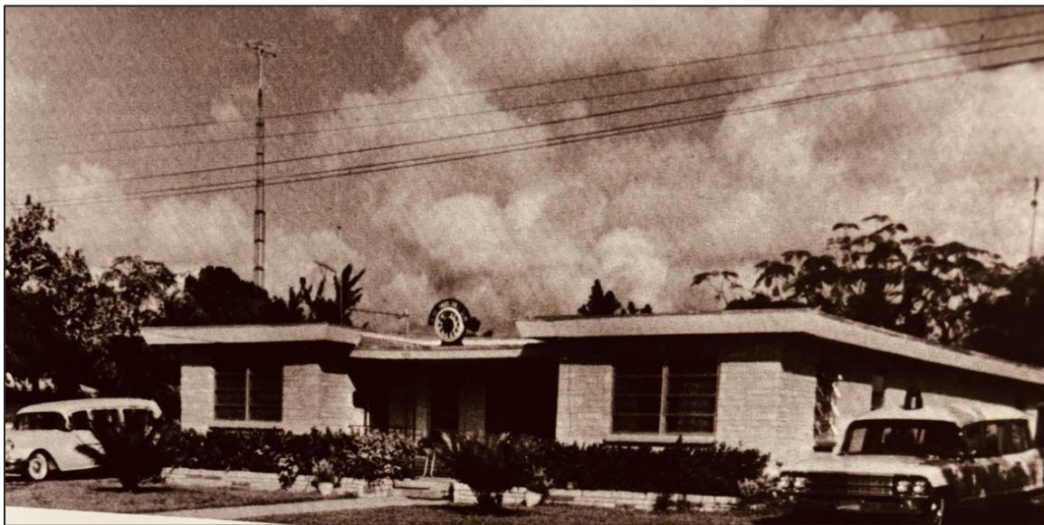
Figure 44. Percy S. Peek Funeral Home at 728 Avenue D (8SL03697), south and east elevations, looking northwest, ca. 1960s.
