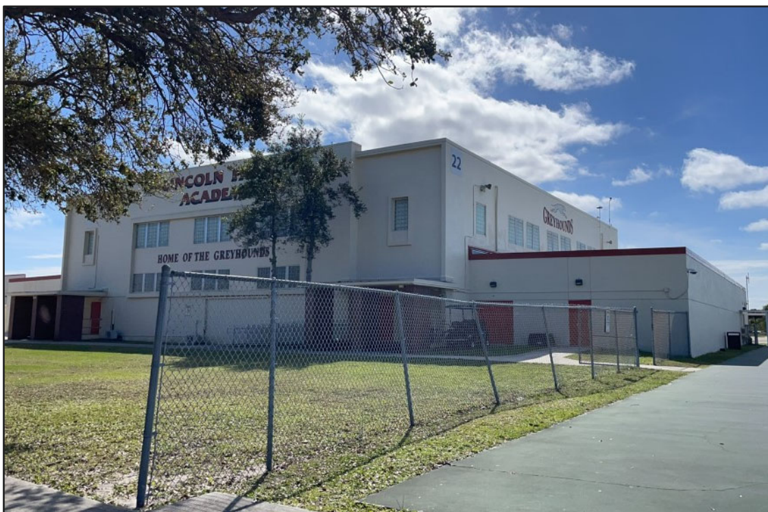
Figure 16. Example of an International style building within the survey area is the Gymnasium at Lincoln Park Academy at 1801 Avenue I (8SL03443).
