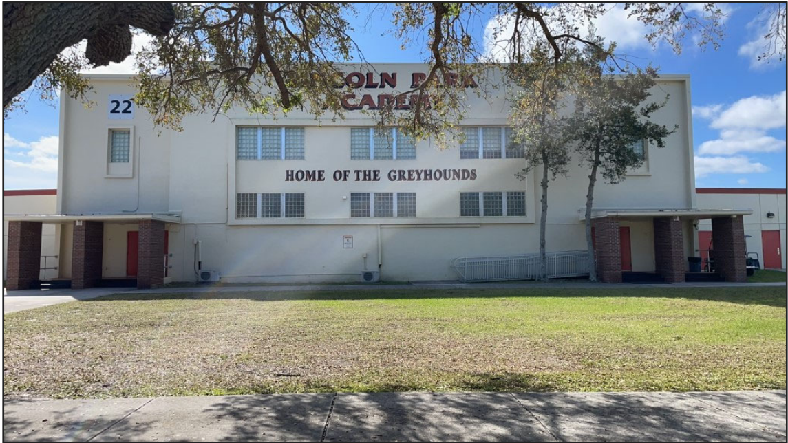
Figure 32. The Gymnasium at Lincoln Park Academy at 1801 Avenue I (8SL03443), north elevation, looking south.
