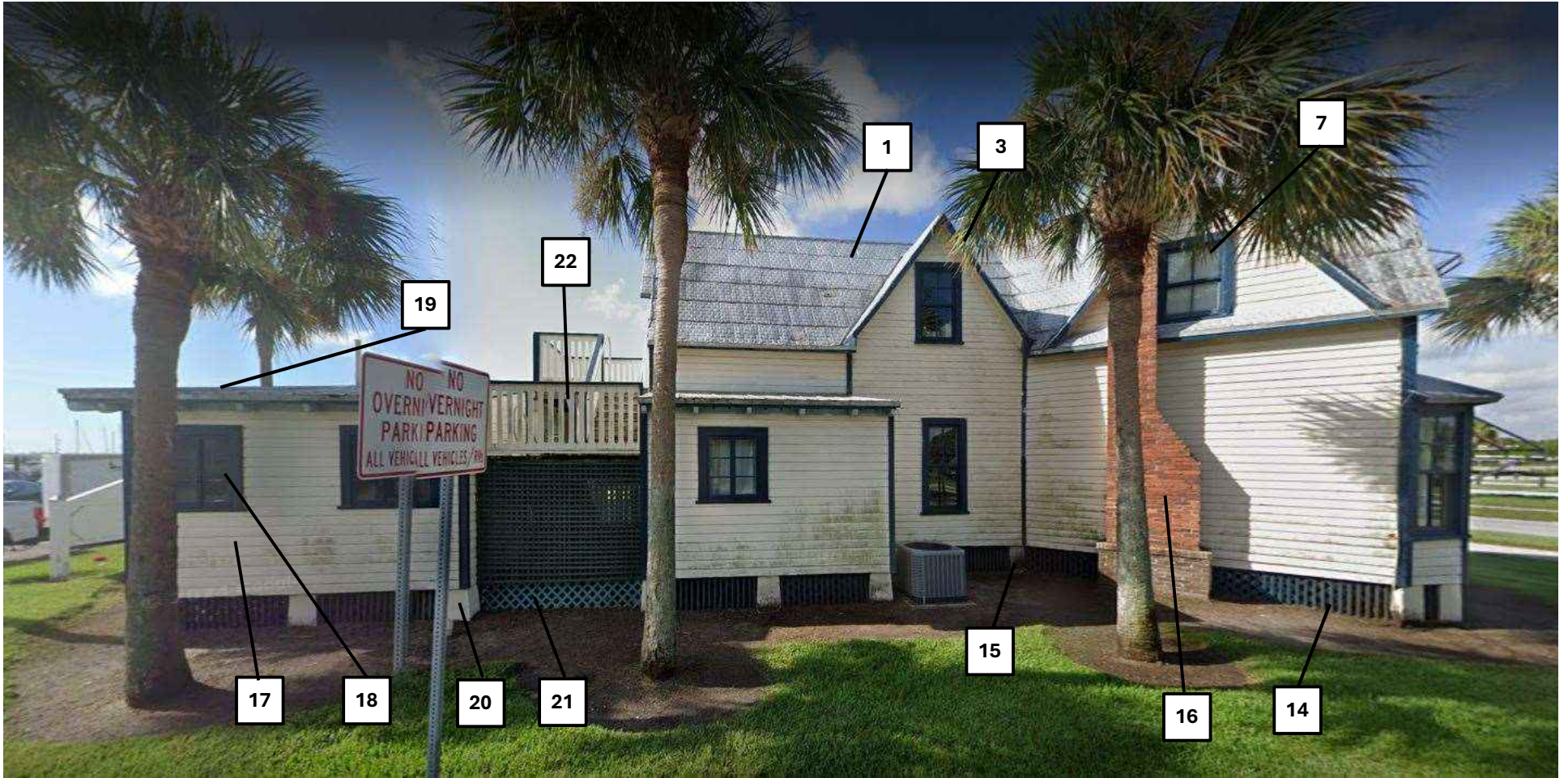
Seven Gables Exterior Rehabilitation North Elevation
