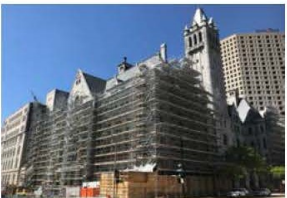
Milwaukee Federal Building Milwaukee WI
