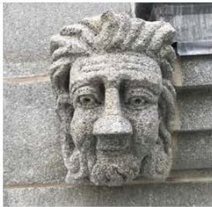
Carved Granite Dutchman Repair to Nose & Mouth
