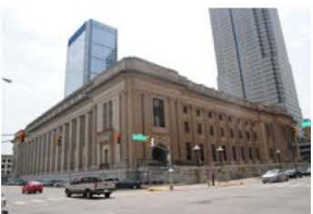
Birch Bayh Federal Courthouse Indianapolis IN
