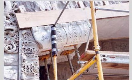
Replacement of Carved Arched Entrance – Wood County Courthouse, Bowling Green OH
