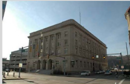
Charleston City Hall, Charleston WV
