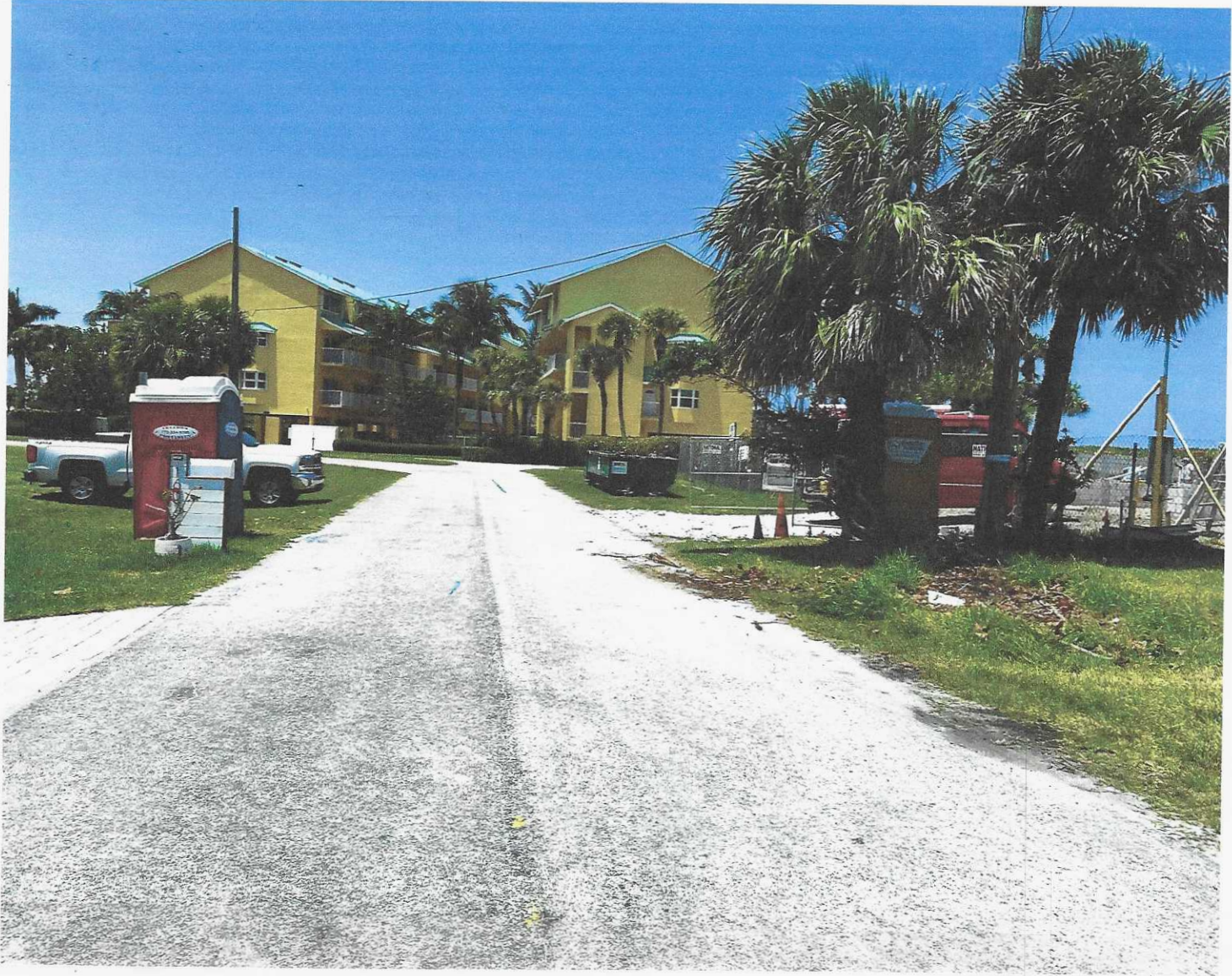
Condominiums located north of 1606 Surfside visible from street at 1606 Surfside Drive
