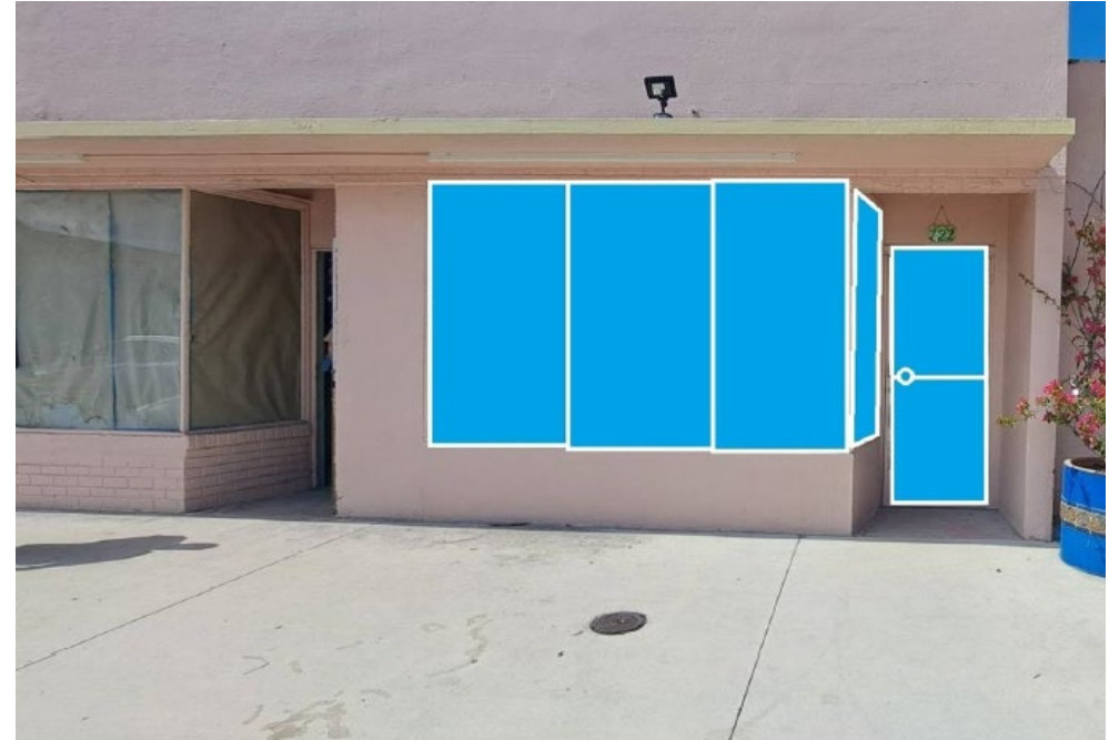
Replace windows and door with impact glass on Unit 722 only
