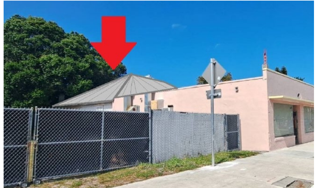
Replace metal roof
