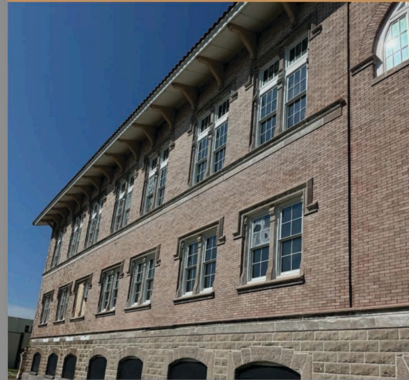
Tuckpointing and Brick Replacement/Rebuilding Complete
