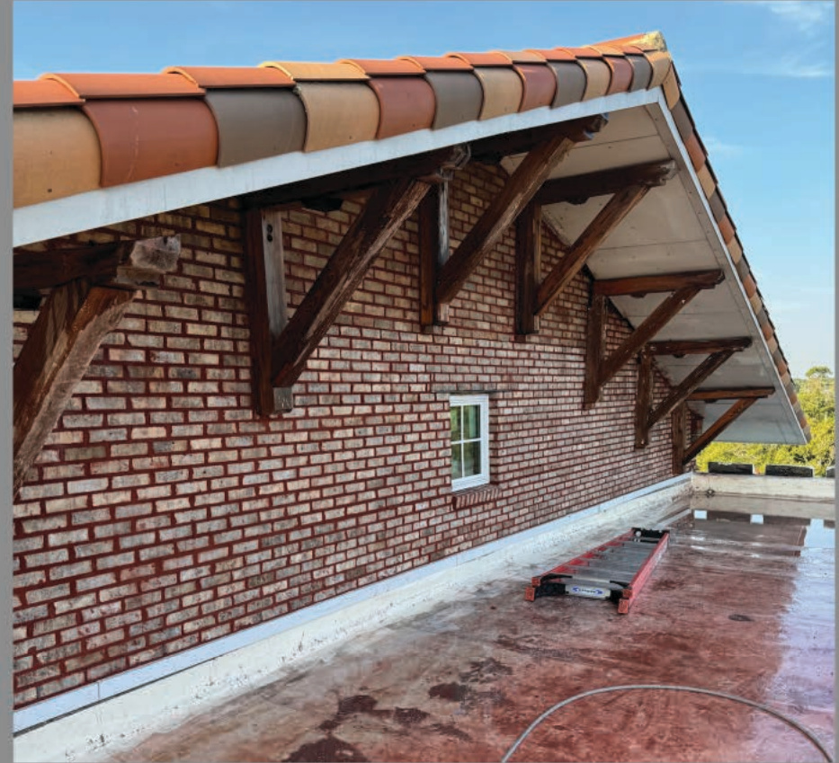
Upper North Brick Rebuilding
