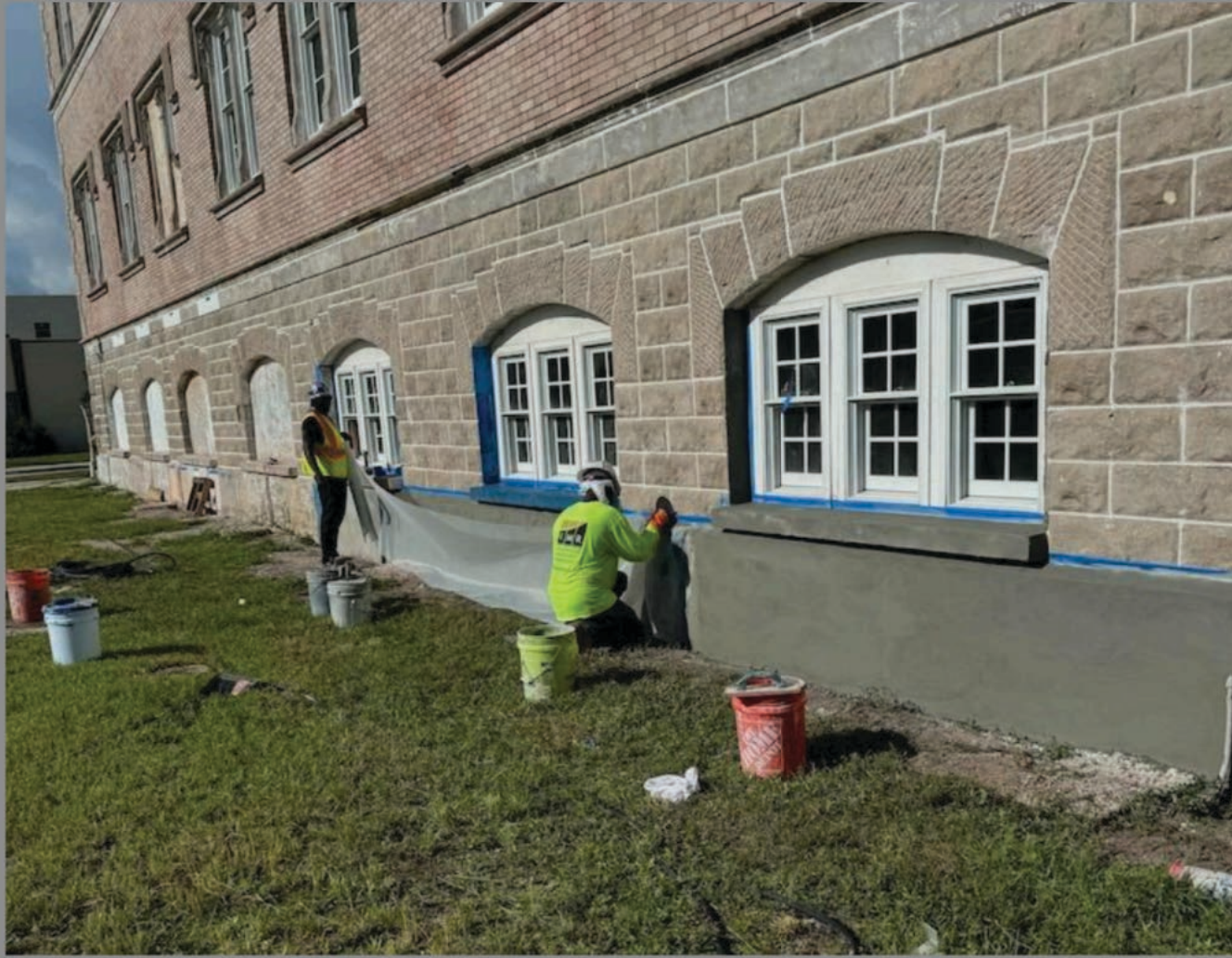
New Stucco System at Concrete Foundation.
