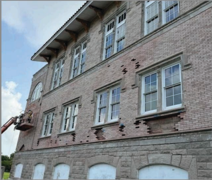
Tuckpointing and Brick Replacement/Rebuilding in Progress
