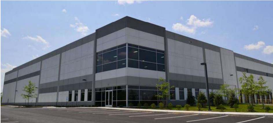
LogistiCenter Exit 8A – Northern NJ
