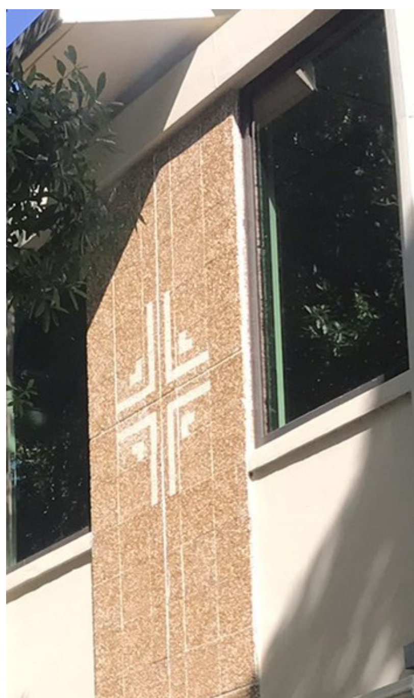
PRECAST CONCRETE TILE MATCH TO EXISTING
