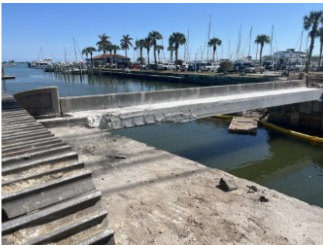
Demolition of the Moore's Creek Bridge
