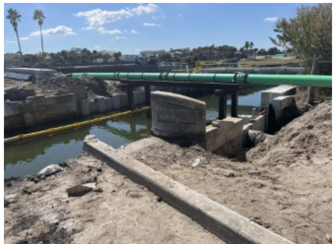
Temporary Support and Forcemain Relocation
