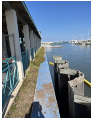
New Seawall Sheeting Panels
