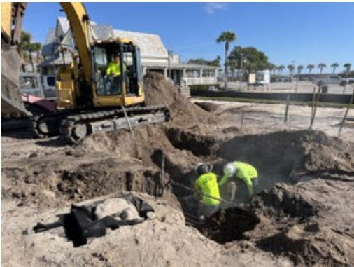
Storm Drainage Construction
