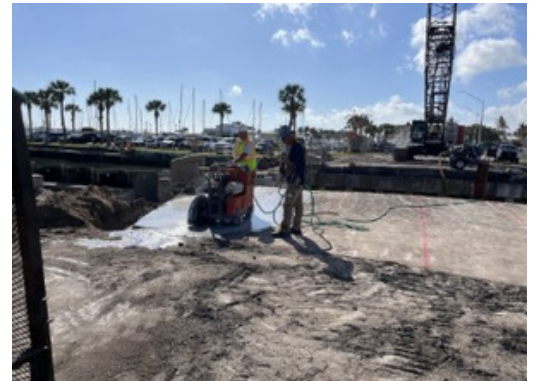
Bridge Deck Removal
