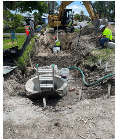
Eucalyptus Drainage Installation
