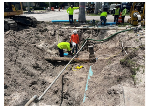
Water Main Utility Upgrades
