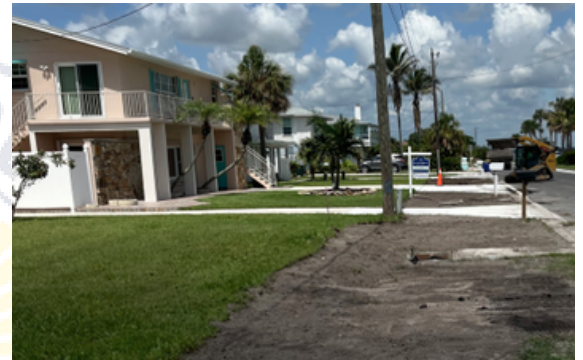
Final Grading for Sod
