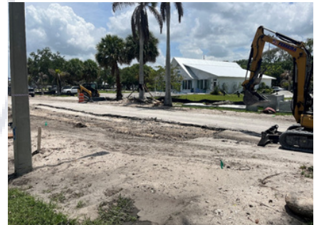
IRD Pavement Demolition
