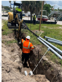
IRD Electrical Relocation Work
