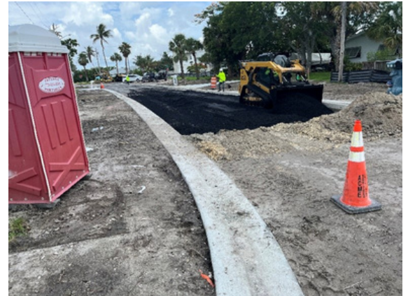
Plover Ave Paving
