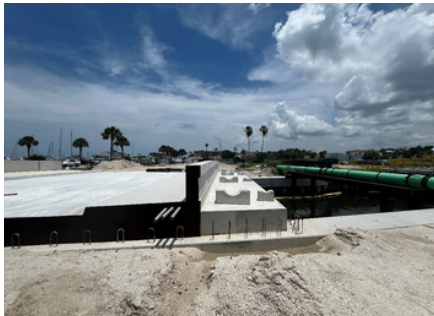
IRD Bridge and Utility Shelf at Moore's Creek
