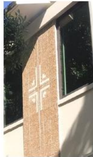
PRECAST CONCRETE TILE MATCH TO EXISTING
