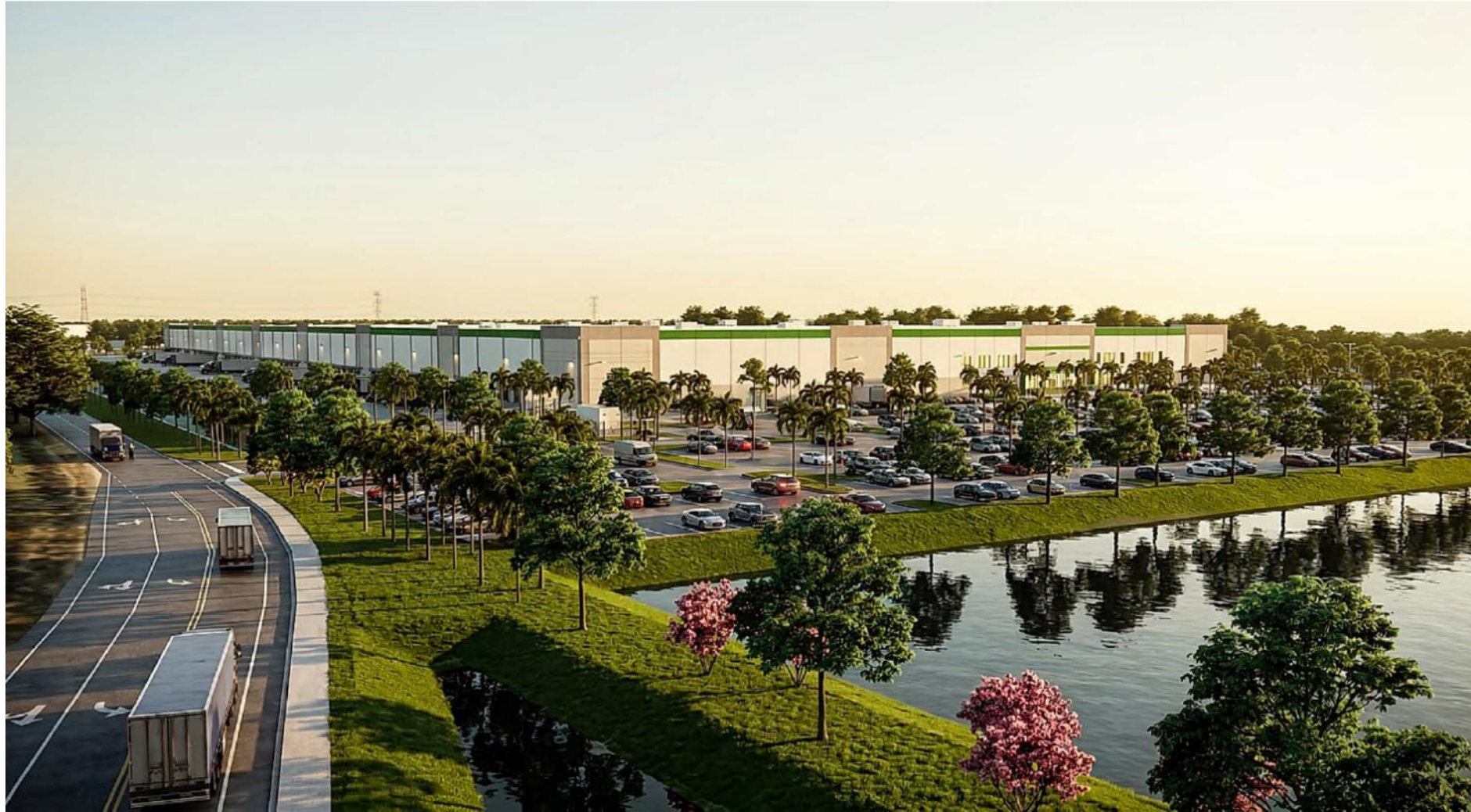
LOOKING SOUTHEAST FROM KINGS HIGHWAY / WHITE ROAD INTERSECTION
