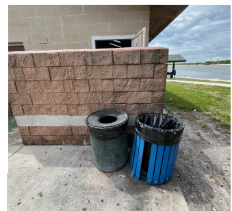
Existing trash receptacles
