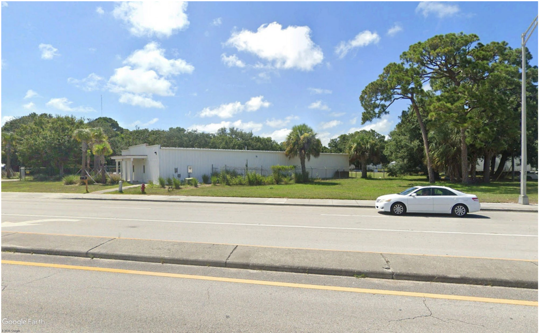
Photo 02 - Looking NW from Okeechobee Road
