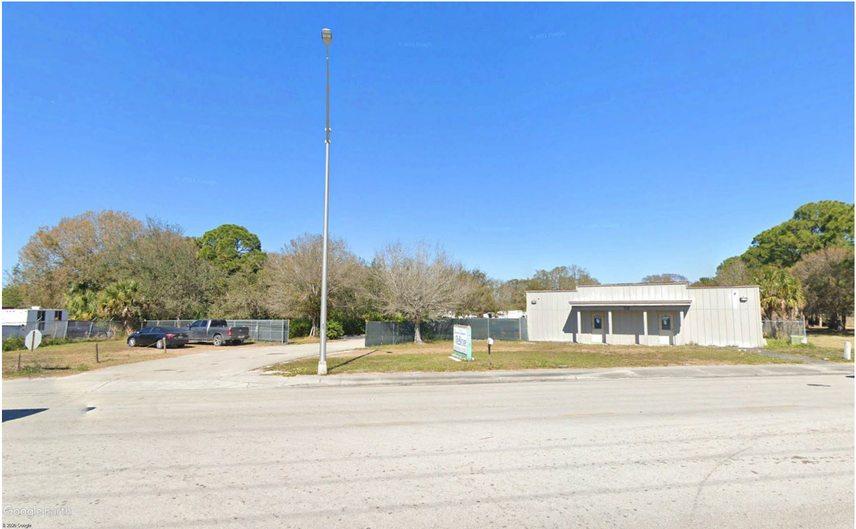
Photo 01 – Looking N from Okeechobee Road
