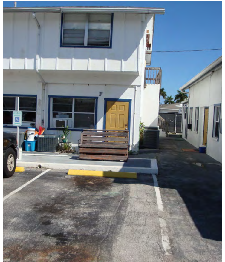
LOOKING EAST AT 2 STORY APARTMENT BLDG.
