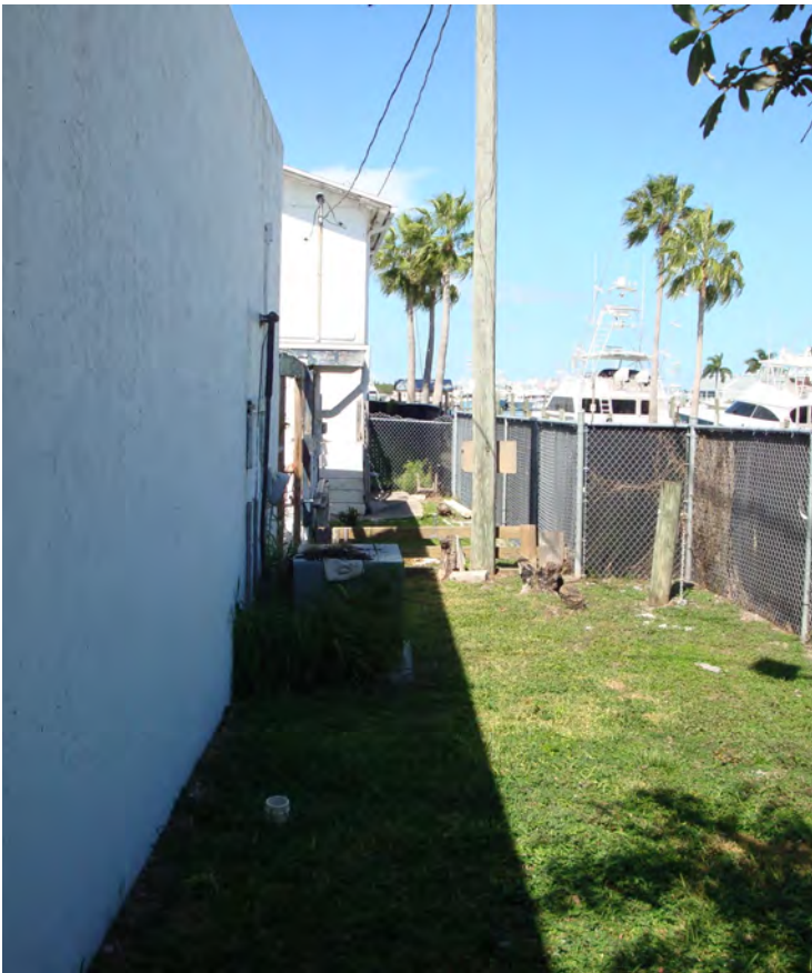
LOOKING NORTH ALONG EAST SIDE OF COMMERCIAL BLDG.
