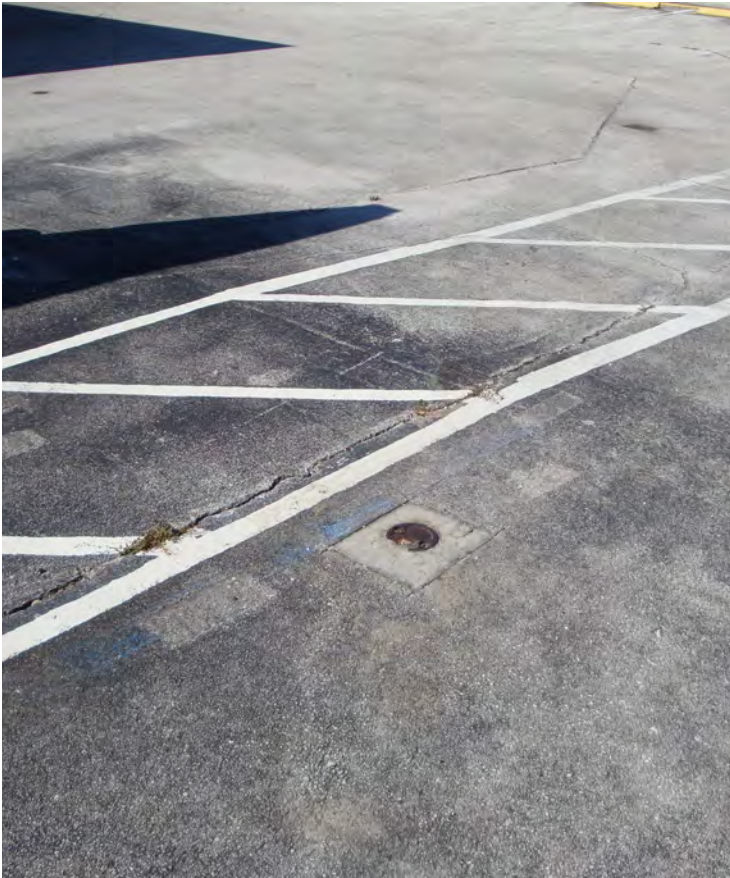
TYPICAL CLOSED MONITORING WELL AT USTs
