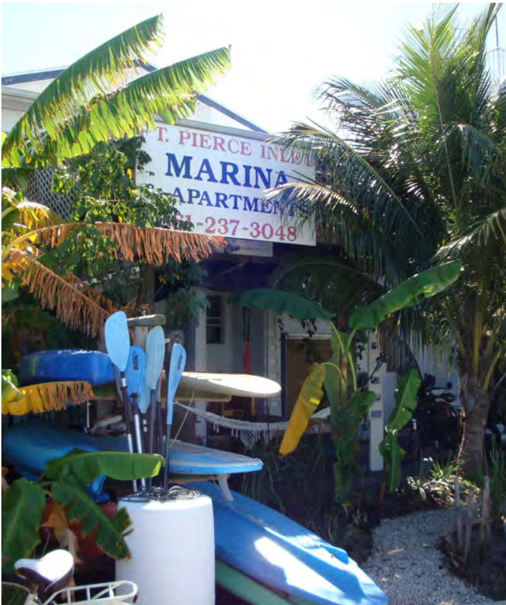
LOOKING SW AT MARINA BLDG.
