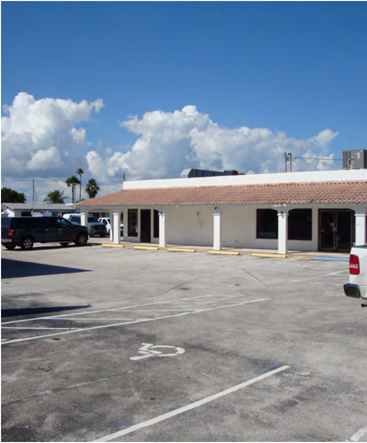
LOOKING NW AT COMMERCIAL BLDG.
