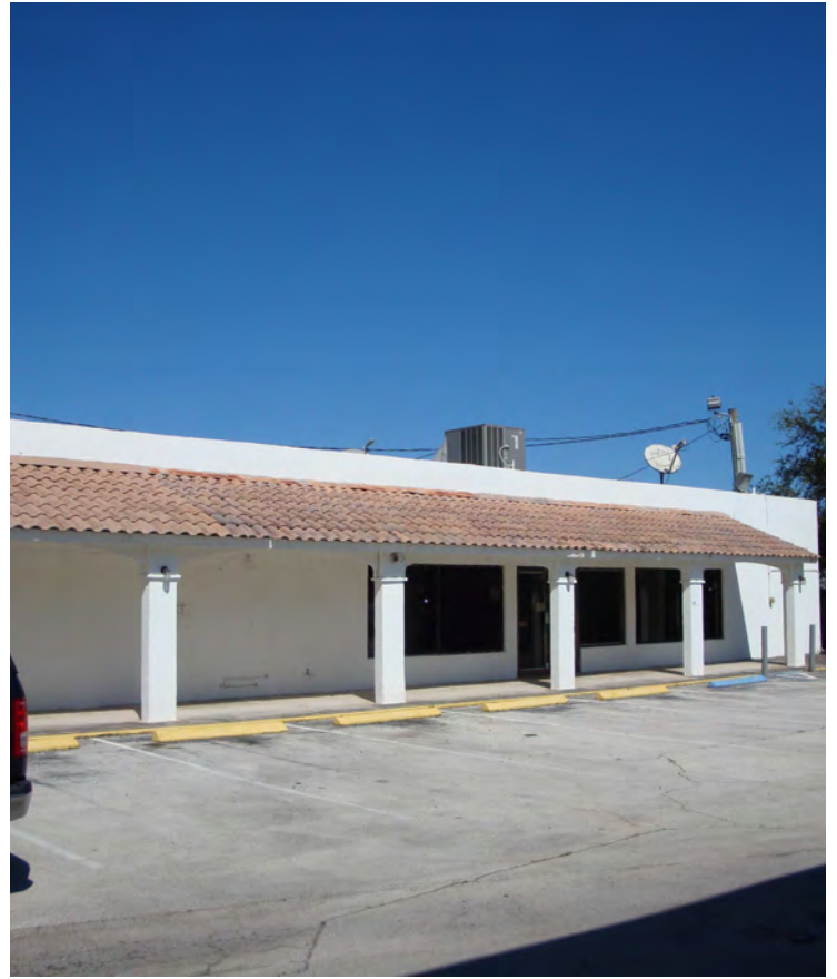
LOOKING NE AT COMMERCIAL BLDG.
