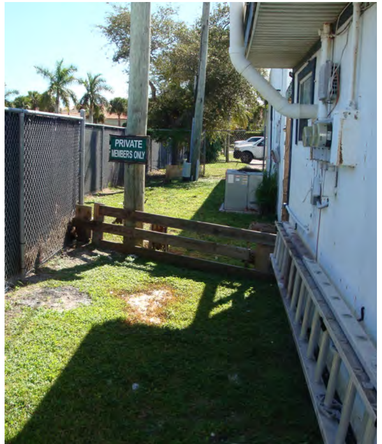
LOOKING SOUTH ALONG EAST SIDE OF 2 STORY APARTMENT BLDG.
