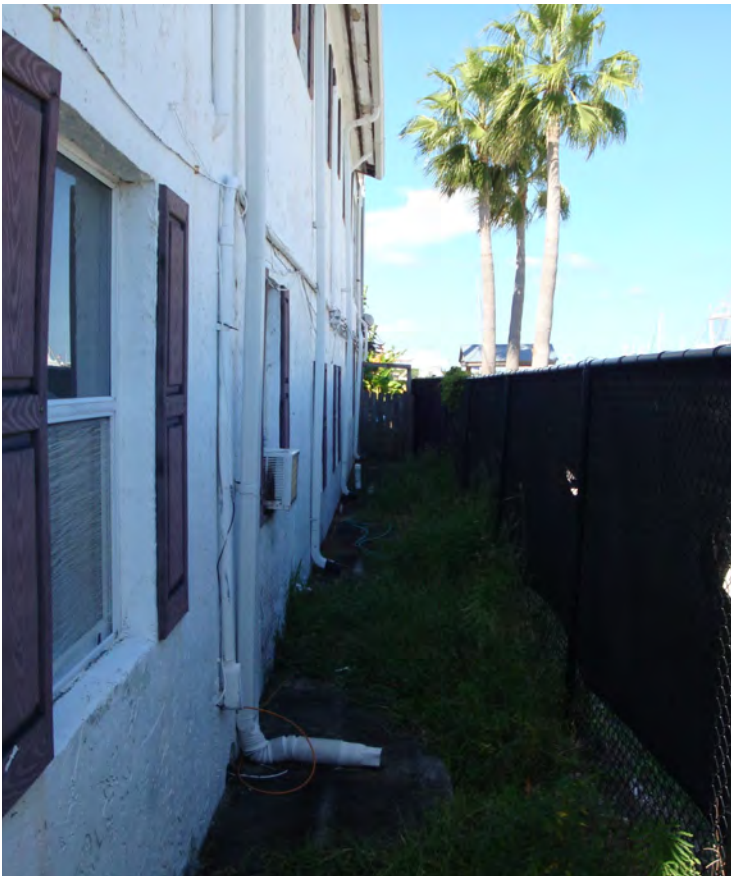
LOOKING NORTH ALONG EAST SIDE OF 2 STORY APARTMENT BLDG.
