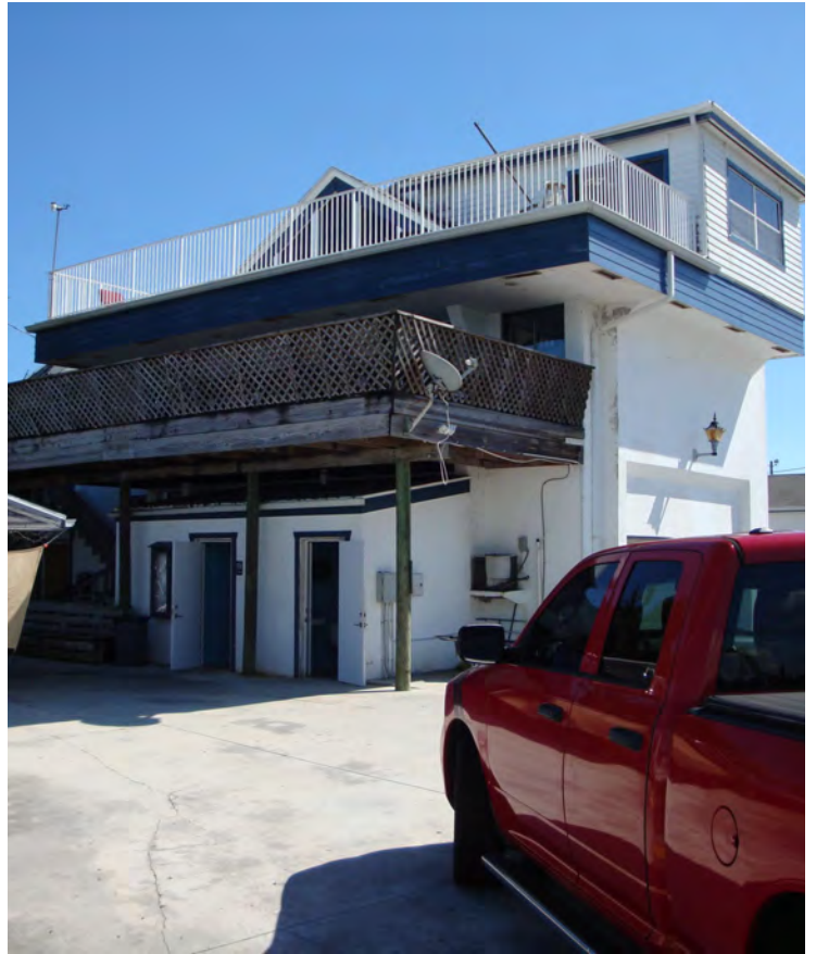
LOOKING SE AT GARAGE BLDG.
