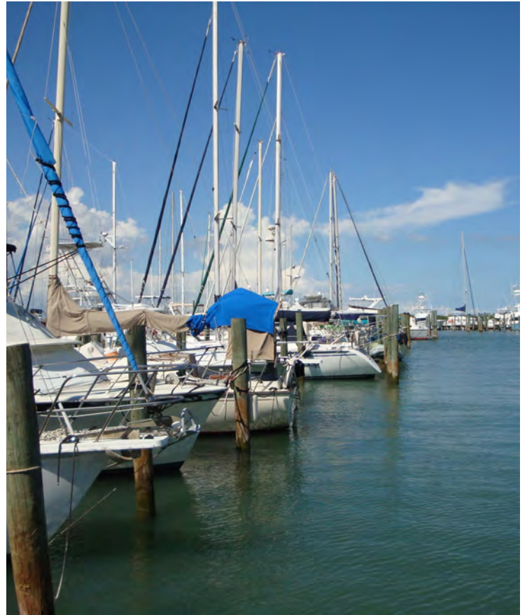
LOOKING NORTH AT MARINA
