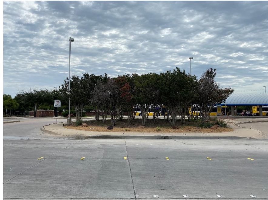
View from the site looking East across North Fifth Street
