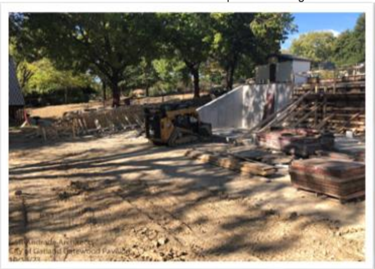
Gatewood Pavilion – construction progress
