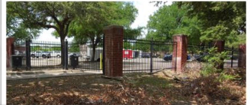
Perimeter Fence pre-construction
