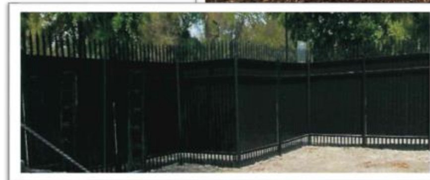
Perimeter Fence – construction progress photo
