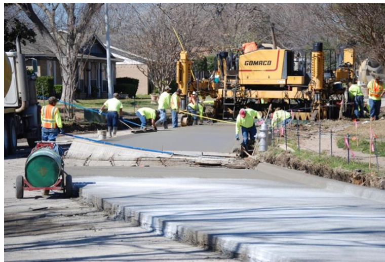
Slipform Paving Operation
