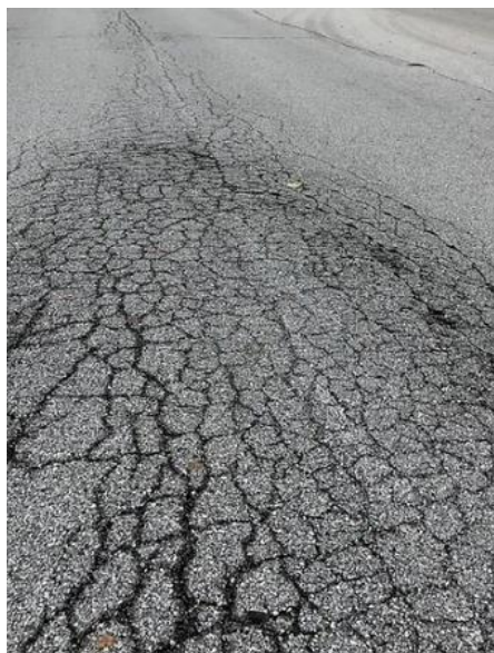
Alligator Cracking
