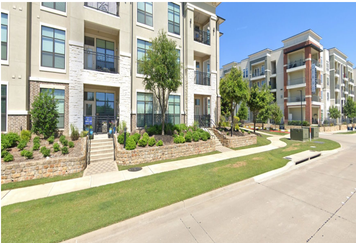
View of west side of Campbell Road, north of Ferris - Multi-Family Residential
