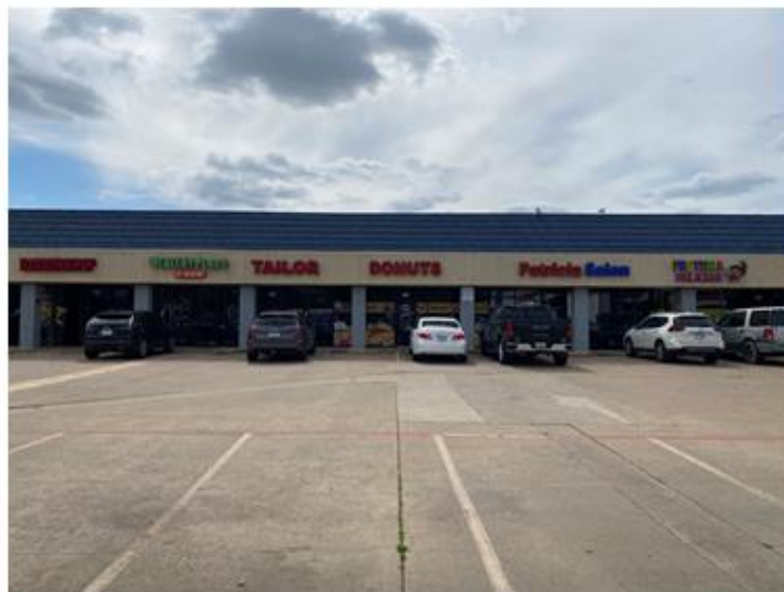
View of the subject property looking West from Broadway Boulevard
