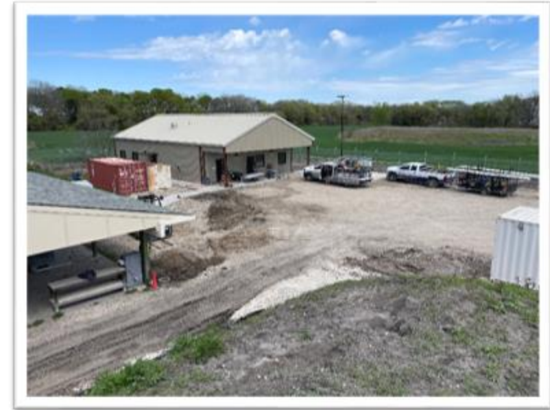
Range - construction progress photo
