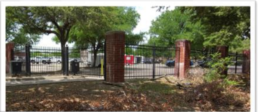
Perimeter Fence pre-construction
