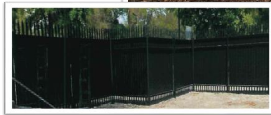
Perimeter Fence – construction progress photo
