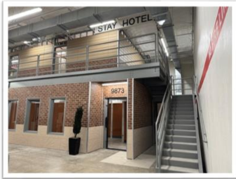
RBT - construction progress photo
