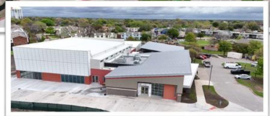
Construction progress photos
