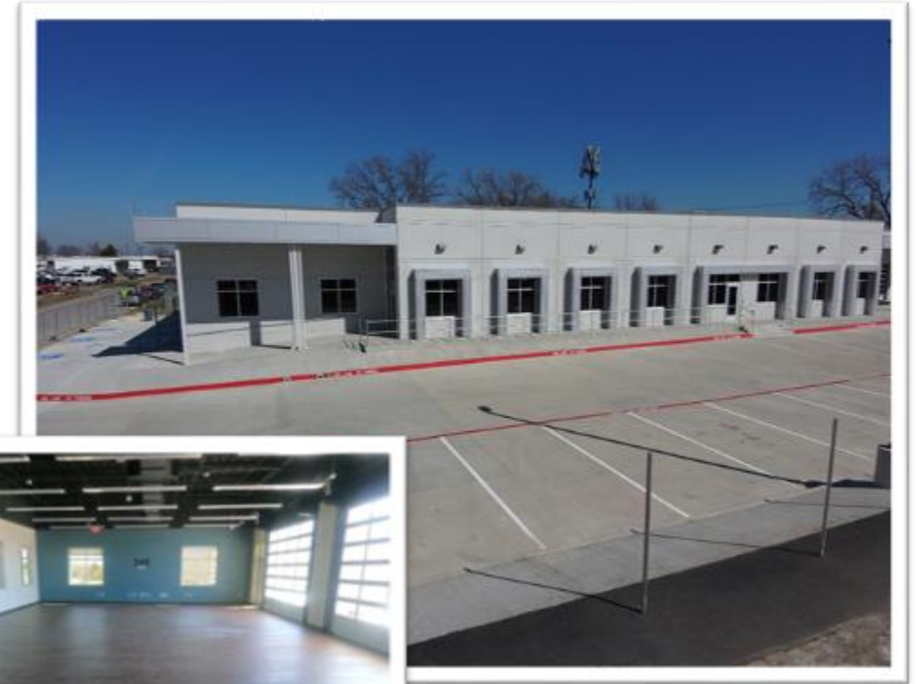
Construction progress photo of new facility
