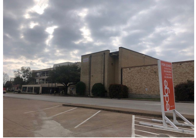
South of the subject property
