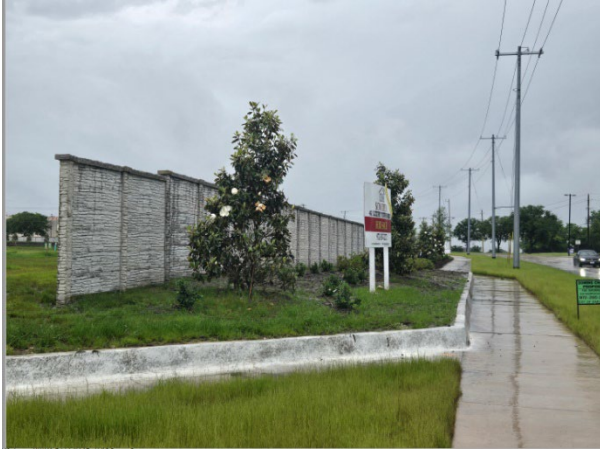
Photo on Roan Road facing north
