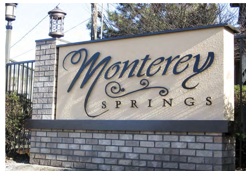
Utilizing CMU Blocks as the Base
