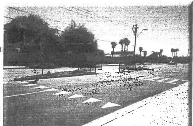
The Pedestrian Refuge Island adjacent to Peoria High School was rebuilt twice after errant drivers destroyed the first two.
