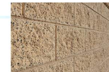
SPLIT FACE CMU
