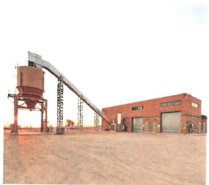
Ocotillo Water Treatment Facility
