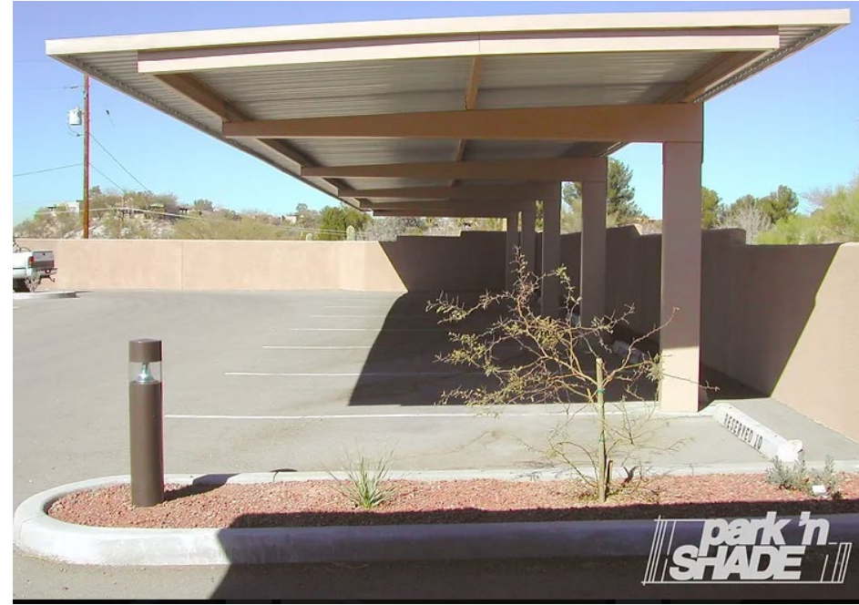
Non-Solar Shade Structure with Cantilever Beam
