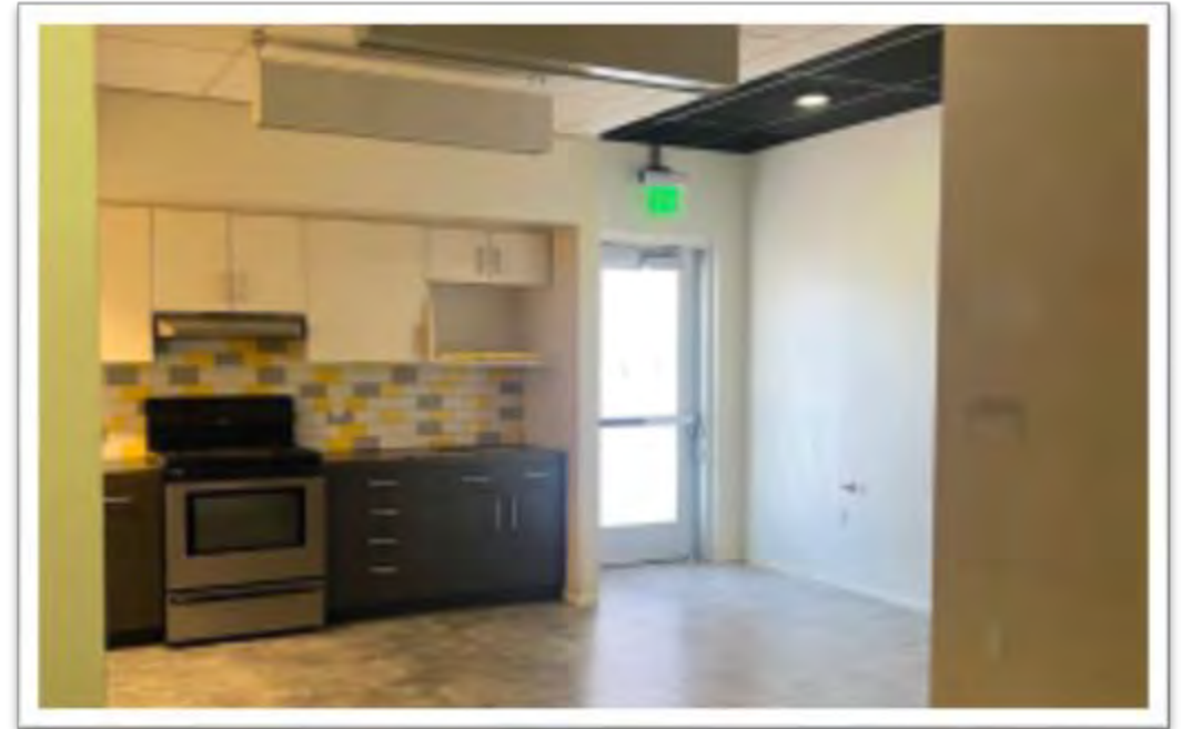
Fiber, plumbing, electrical
