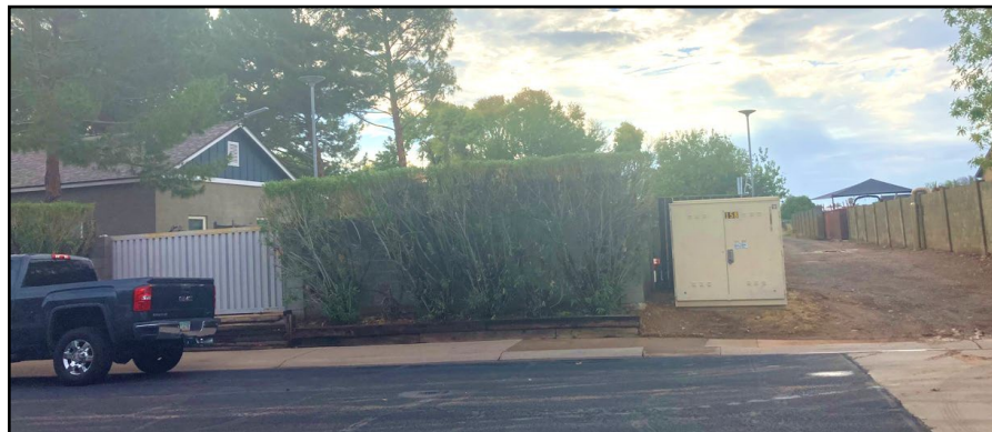
View of side yard from 53rd Avenue. Looking east.
