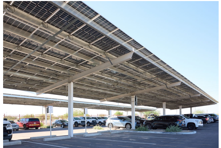
GRPSTC West Carport
