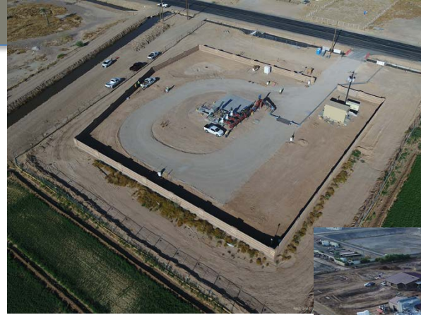
Raw Water Pump Station
