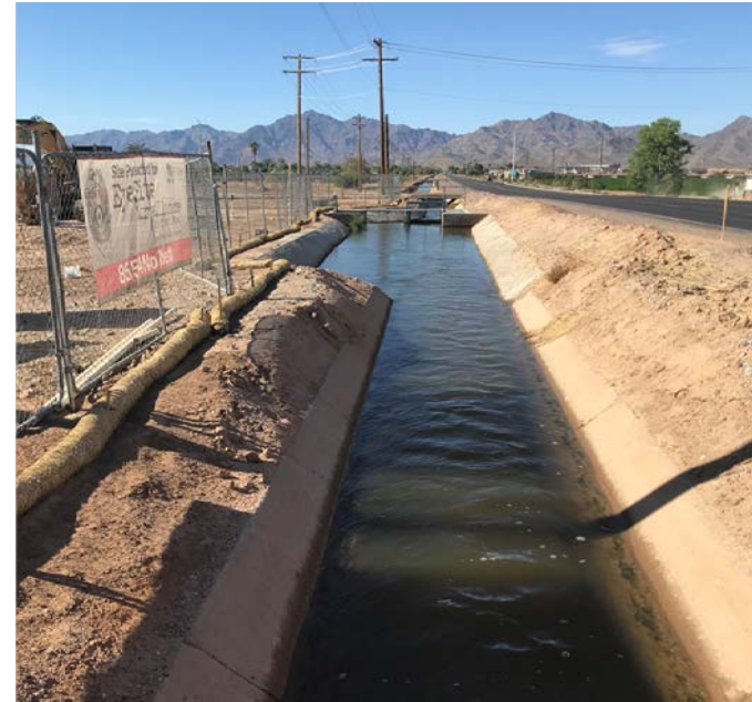
SRP Turnout to Raw Water Pump Station
