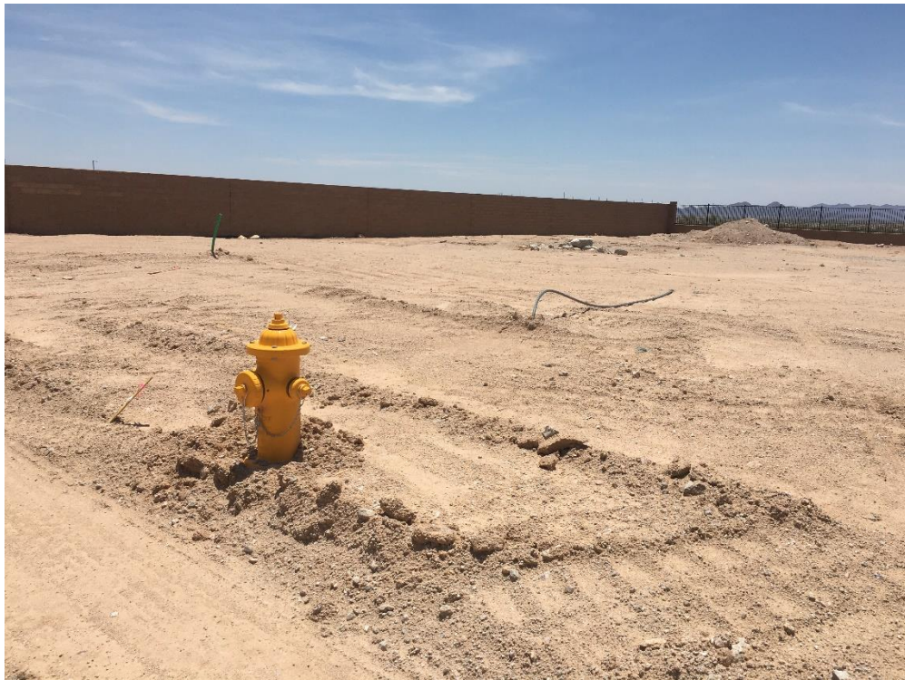
This fire hydrant reflects the finished condition of underground water and sewer lines.
