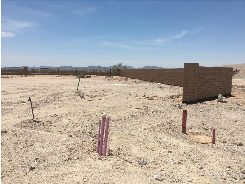
Another view of mostly finished perimeter slump block wall and wrought iron the fence.
