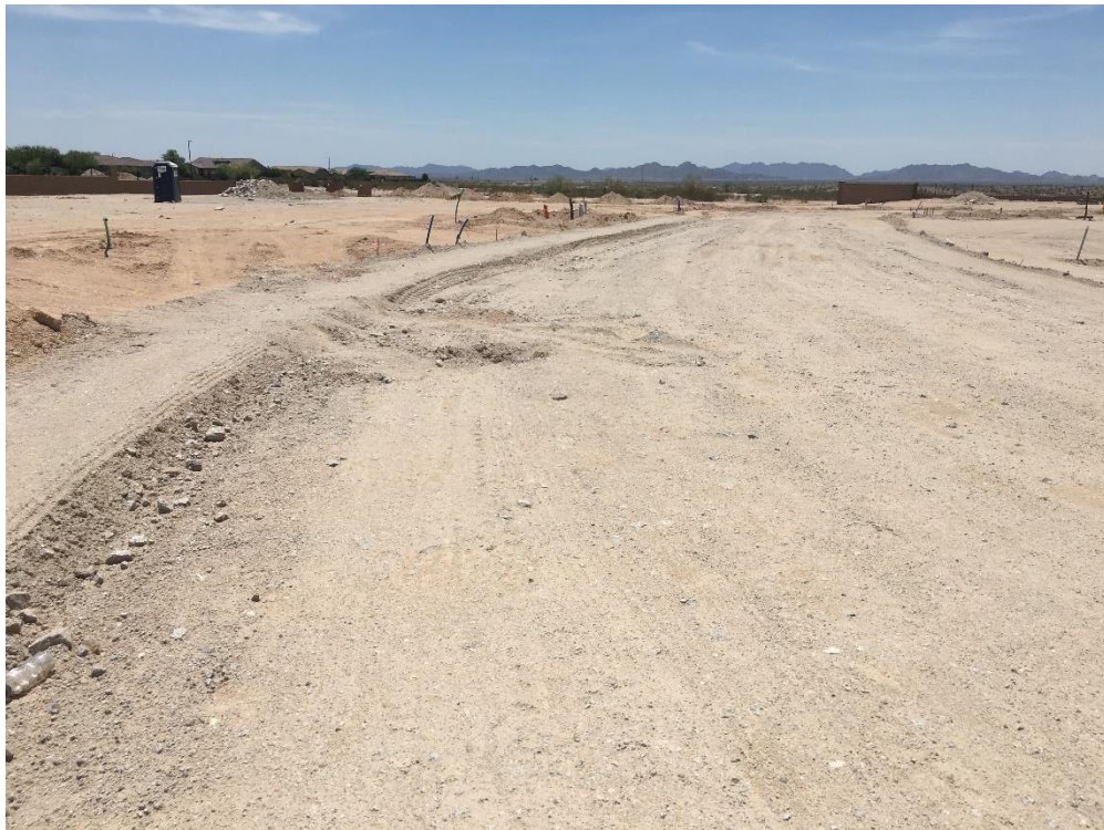
Another mostly graded interior street.
