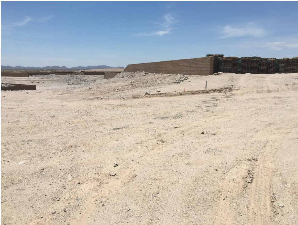
Much of the perimeter concrete block walls have already been constructed.
