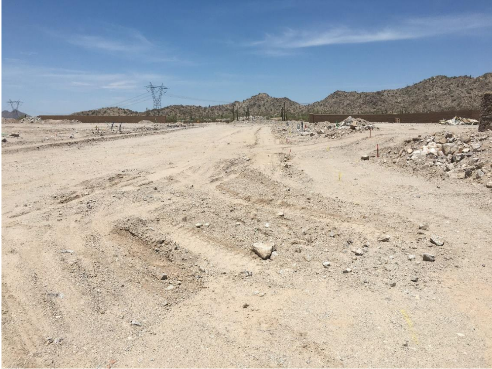
Looking west over graded interior street and lot pads.
