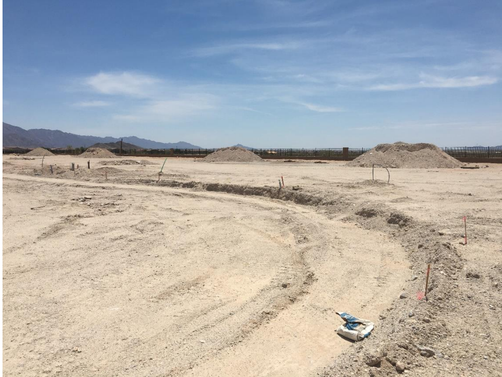
Looking southeast from near the west end of the property.
