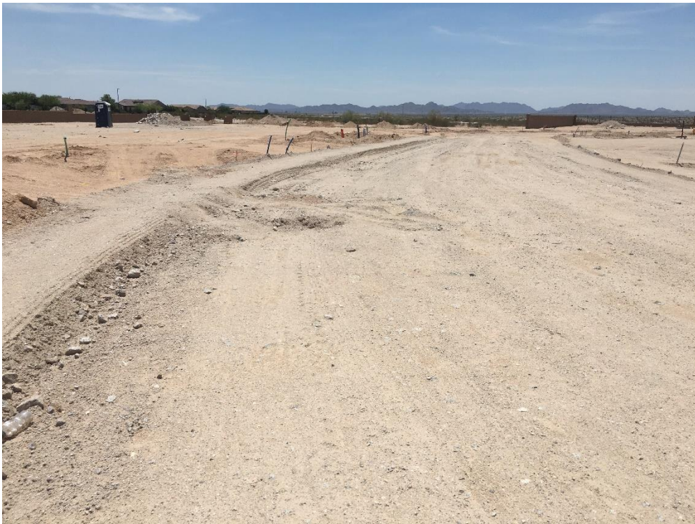
Another mostly graded interior street.
