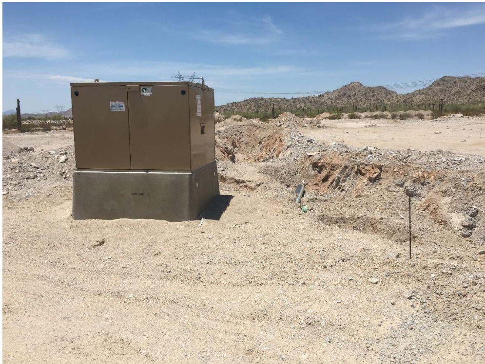
View of underground utility box and related trenching.
