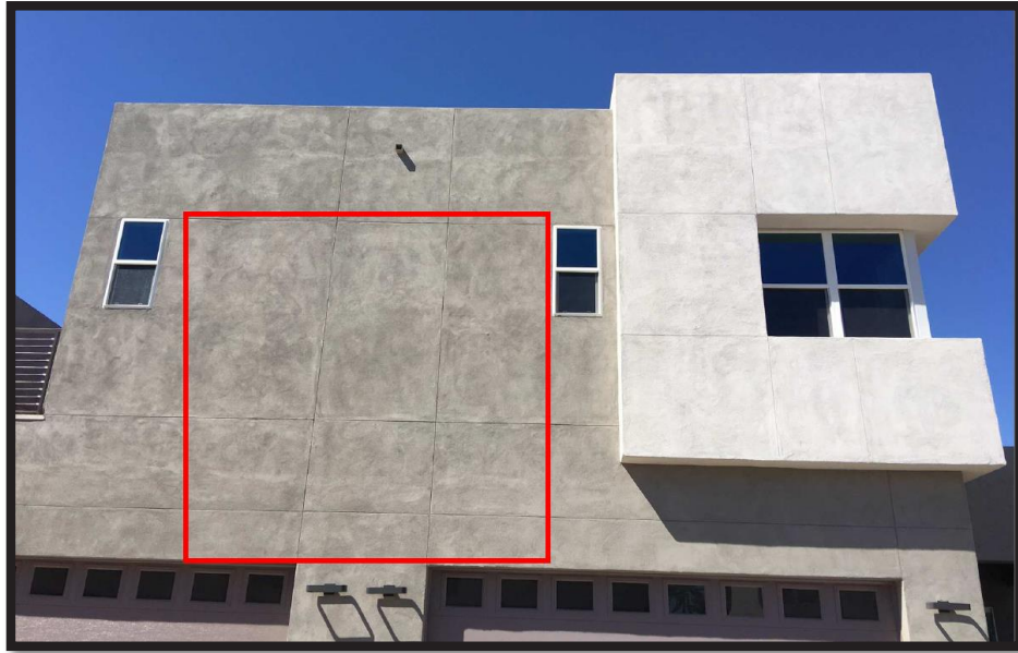
Horizontal and/or vertical stucco control joints
