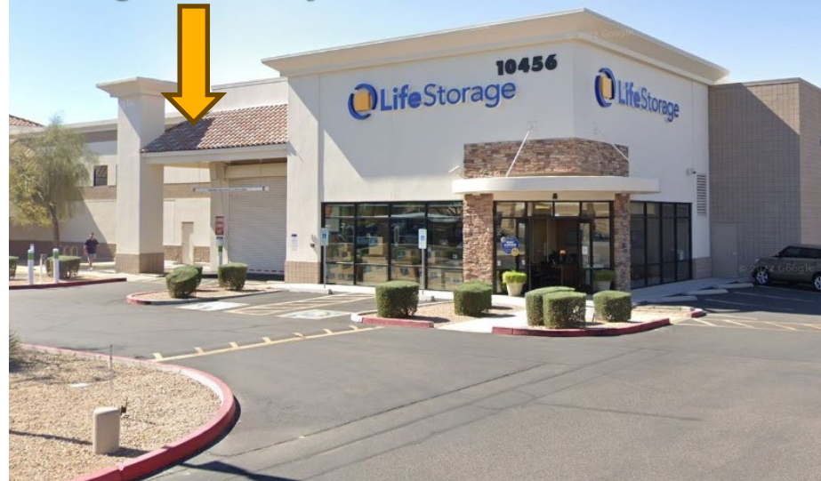
Garage door entry
