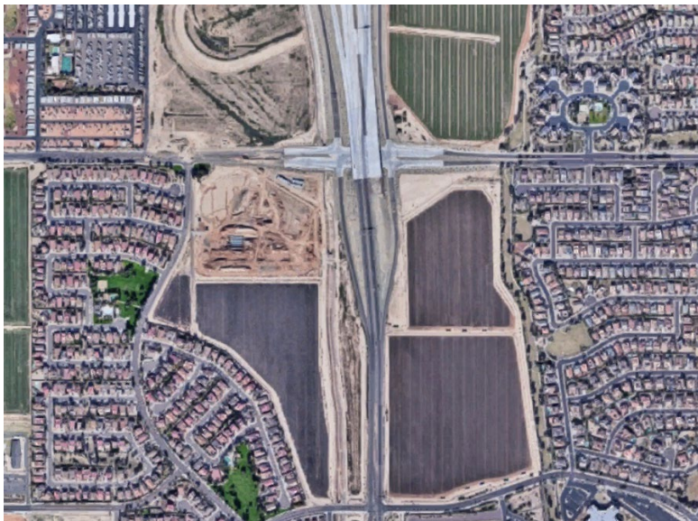
The terminus of AZ-303. Additional right of way for the highway's expansion is evident.
