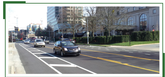
Buffered bicycle lanes provide extra space between bicycles and motor vehicles.
